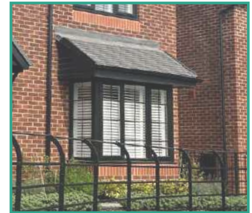
Bay paned window with dark window frame
