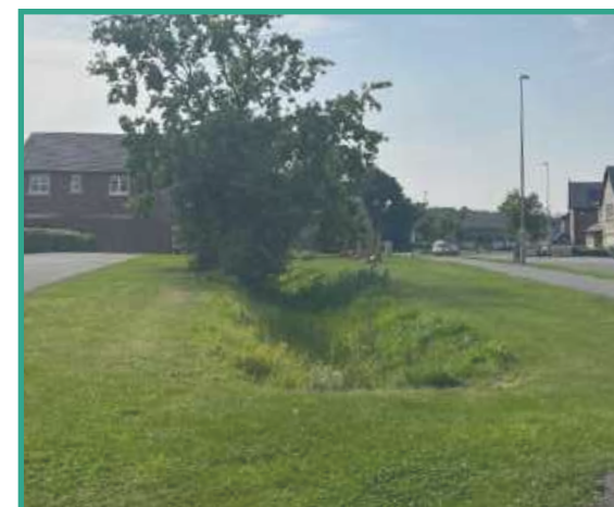
Swale SuDS - providing flood mitigation, accessible green space and acting as natural buffer within a large housing estate
