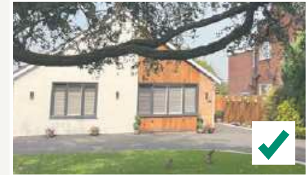
Updated facade with render, timber cladding and new windows
