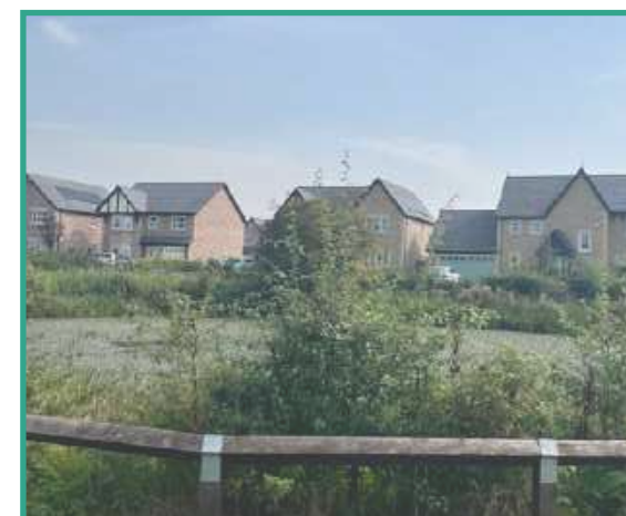
Drainage pond SuDS - providing landmark space, flood mitigation and an attractive natural feature of the housing estate
