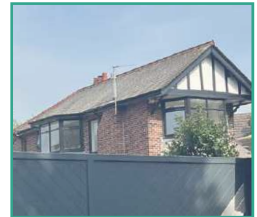
Box gable with clay ridge tiles, timber bargeboard and timber corbel
