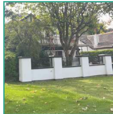
White rendered wall and wall posts with metal fence detailing
