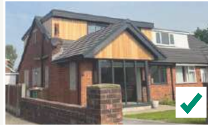
Updated facade (left) and original 1970s facade (right)
