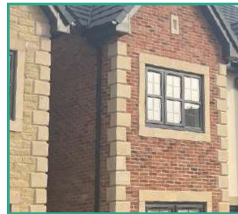
Stone window headers, window cills and quoining
