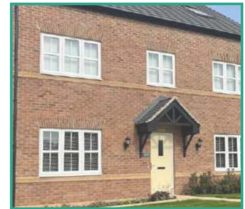
Red brick window headers and brick course lines
