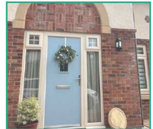
Centrally located doorway with side windows and brick/stone surround
