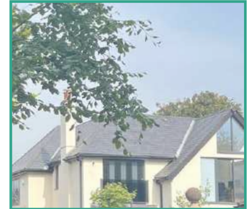
Hip roof with projecting gable to the front elevation creating variety
