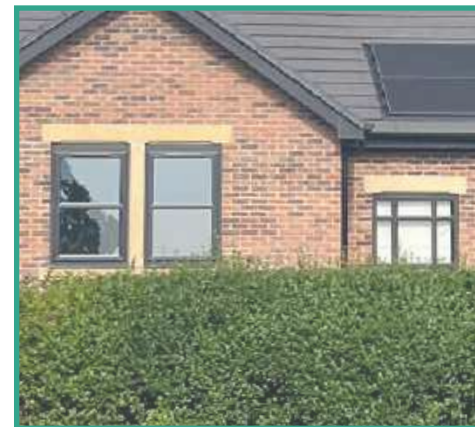
Anthracite framed windows with stone headers, cills and mullions
