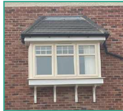
Oriel window with imitation paned sash windows
