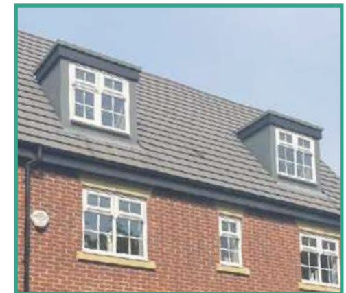
Imitation paned sash windows with dormer windows projecting from roof
