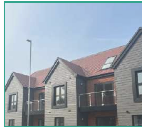
Projecting gables creating interest and variation in the building frontage
