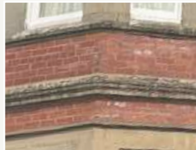
Masonry course line
