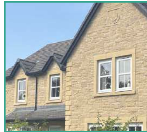
Stone window surrounds, date stone and stone quoining
