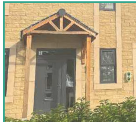
Imitation timber door with timber and grey slate projecting porch canopy
