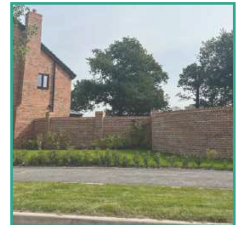
Red brick wall and wall posts with grass buffer and hedging to define boundary between private front garden and public realm
